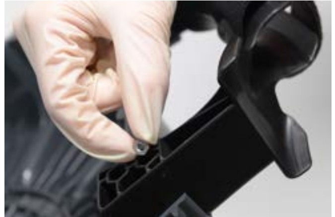
Figure 25 – Place nuts into screw holes
