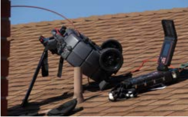
Figure 5 – Positioning for rooftop inspections
